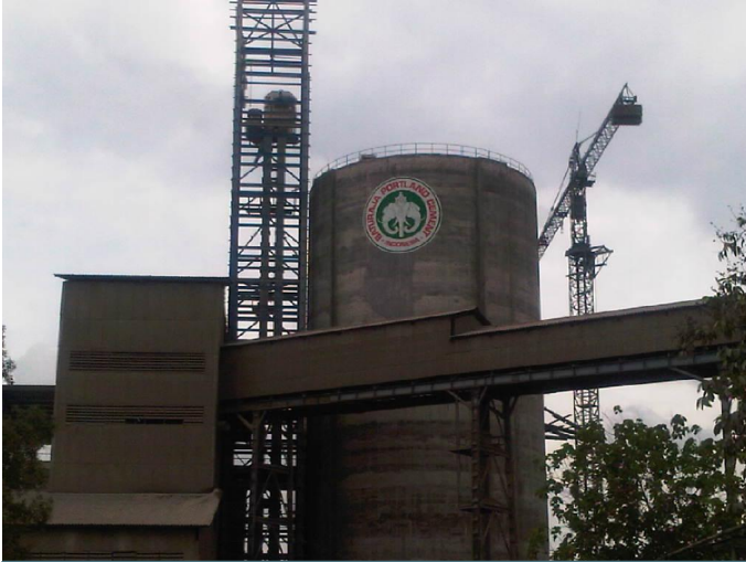
Cement Mill & Packer PT Semen Baturaja
