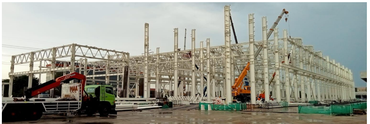
Konstruksi Baja Depo LRT JABODEBEK Light Maintenance Building PT. Adhi Karya
