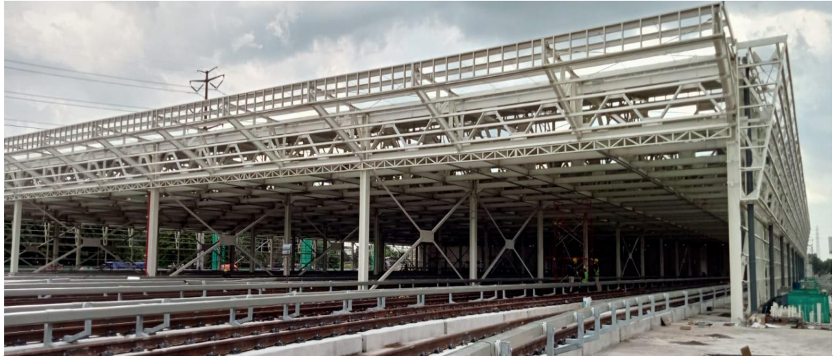
Konstruksi Baja Depo LRT JABODEBEK Stabling Building PT. Adhi Karya
