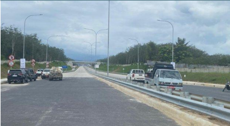
Guardrail Tol Trans Sumatera Tebingtinggi - Serbalawan
